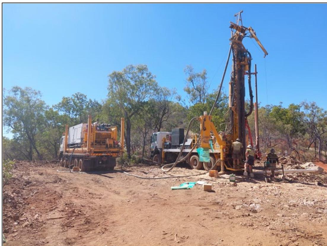
*Figure 8: RC Rig Drilling at the Project during 2023*
